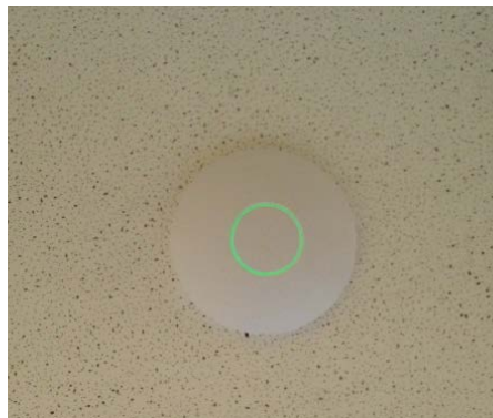
Fig. 2. AP point installed on campus building.
