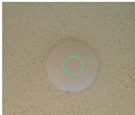
Fig. 2. AP point installed on campus building.
